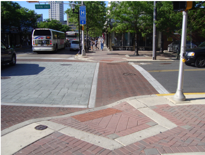
Figure 3: Enhanced Brick Crosswalks
