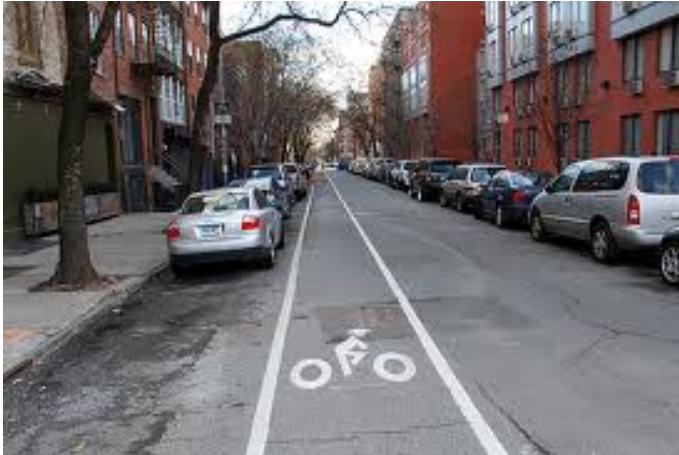
Figure 14: Left-Side Bicycle Lane
