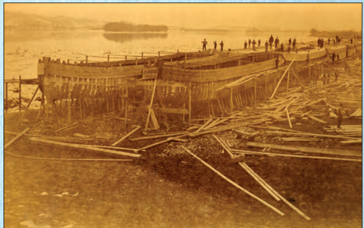
Workers stand along the tops of two long rows of canal boats and along the side of wooden scaffolding during construction in Highspire, circa 1870. The more than 3,000 miles of roads and 1,200 miles of canal built by the state and private companies between the 1790s and 1860 were part of a transportation revolution that sped the interchange of coal, lumber, food products, and other materials in Pennsylvania's booming economy.
